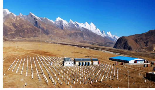
(b) ARGO-YBJ is a Chinese-Italian experiment located at Tibet, to observe very high energy gamma rays using an extensive air-shower array consisting of a carpet of RPCs.
