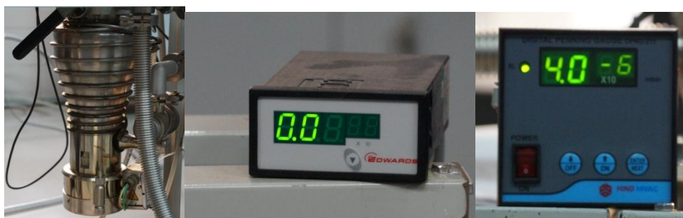
Fig. 2.4. (L-R) Diffusion pump, Pirani Gauge and Penning Gauge readouts
